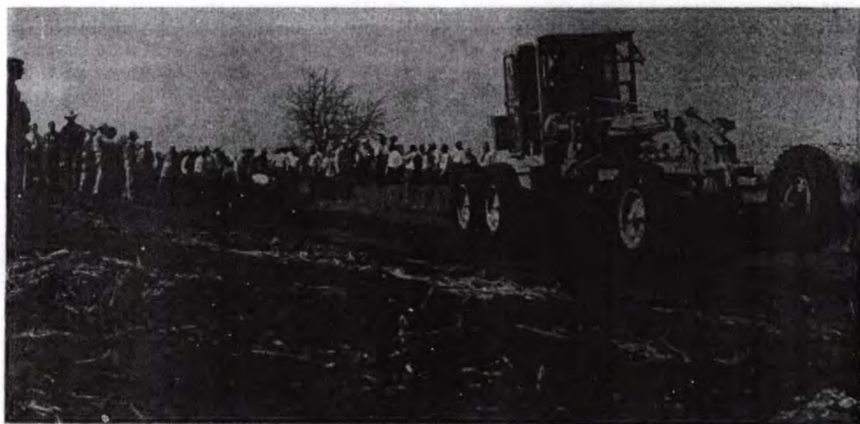
Constructing a broad base terrace as a part of the small watershed demonstration near Rose Hill, Kans.
